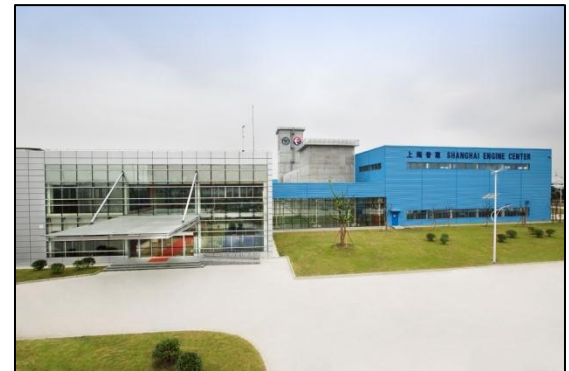
P&W and joint venture partner, China Eastern Airlines, opened an advanced, environmentally friendly CFM56® engine overhaul facility in Qingpu district of Shanghai
