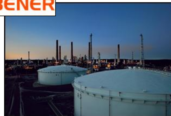
Chubb Ajax (Netherlands) project – complete Fire protection of a new bioethanol factory
