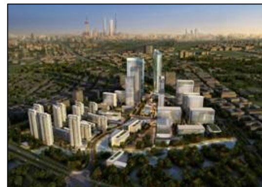
Commercial HVAC win for energy efficient services in Shanghai's New Jianwan District
