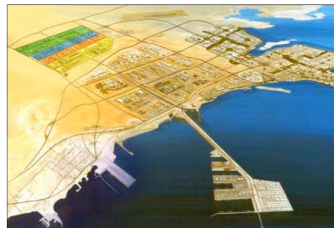
Saudi Kayan project – plastics mfg facility $4M fire and gas safety products
