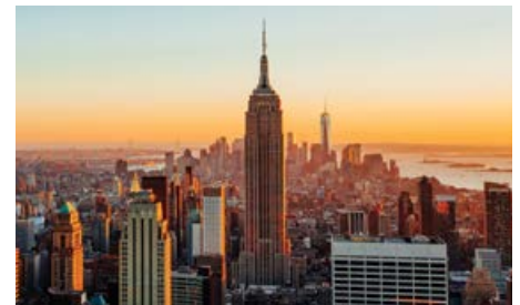
Otis installed the original elevators in The Empire State Building in 1930. More than 80 years later, we are modernizing these elevators as part of an extensive building refurbishment.
