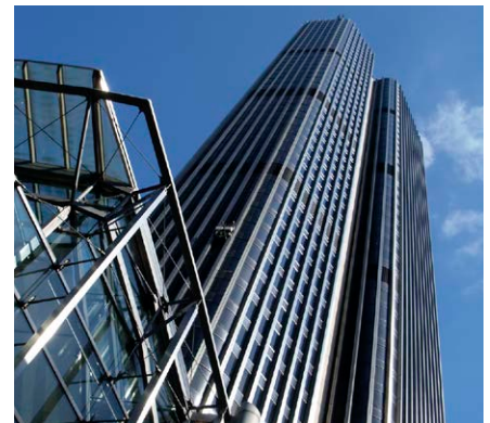
Otis UK recently modernized 25 lifts in Tower 42, London's first skyscraper, first occupied in 1980.
