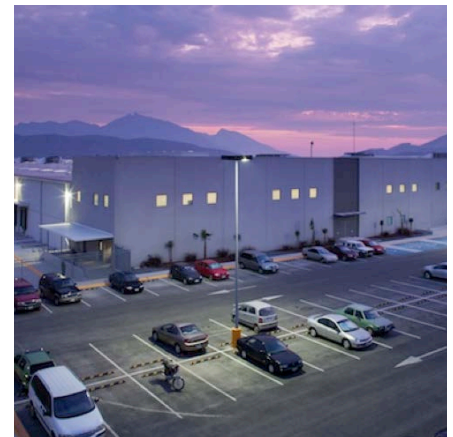
One of Carrier’s facilities in Mexico holds the designation of being the first HVAC factory in the world to earn LEED Gold certification.
