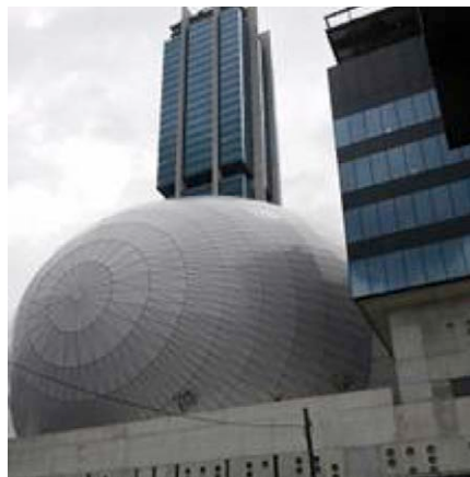
Iconic multi-tenant complex located in Monterrey, comprising a convention center, shopping mall, auditorium, office building and hotel. UTC provided technology for video surveillance, access control, fiber communications, building automation and fire detection.
