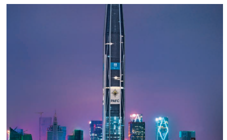
The Ping'An Finance Center, which will be China's second tallest building when completed, is equipped with Otis SkyRise® elevators. UTC Climate, Controls & Security brands, including Carrier, are also providing products and services.
